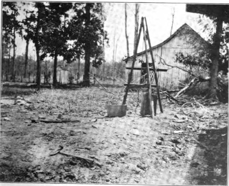
B. A COMMON BUT HIGHLY DANGEROUS WELL LOCATION NEAR BARN AND OUTHOUSES.
